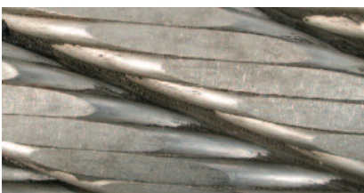
Rope abrasion caused by normal operating condition on a high cycle crane. Rope must be retired.
